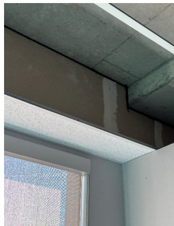
Photograph 6 – Asbestos-containing black tar/caulking.
