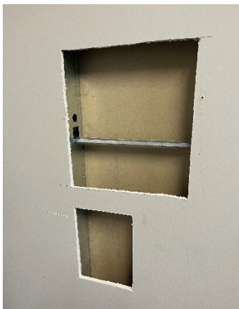
Photograph 5 – Typical space between drywall walls.
